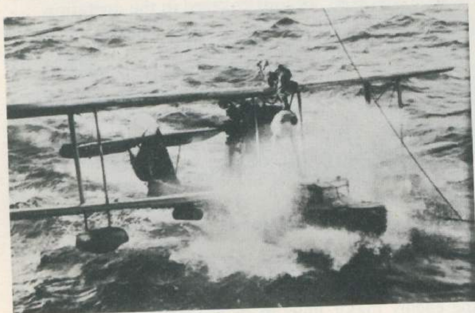
Recovery 4: As the Walrus is raised level with the catapult, heaving lines are thrown across and secured to steady the aircraft as it is swung inboard. The crewman catches one as the pilot secures another.
