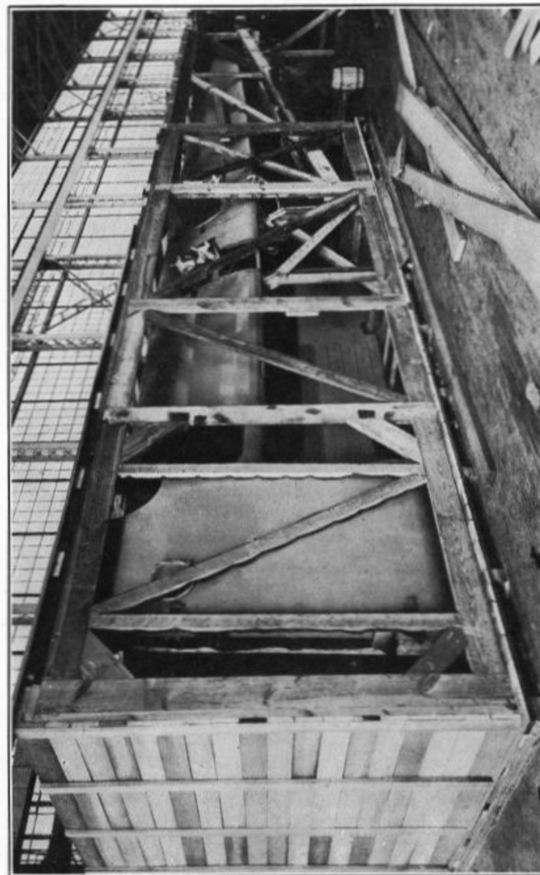
FIG. 20.—HULL IN CASE READY TO BE BOARDED UP.
