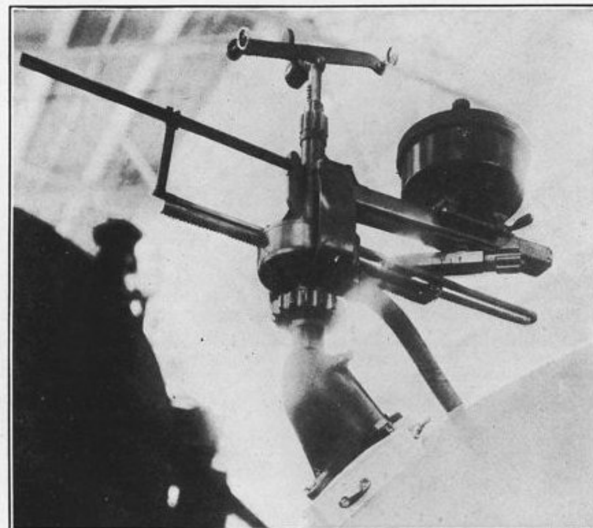
FIG. 49.—SIDE VIEW OF NEW TYPE BOMB SIGHT ATTACHED TO BOW.
