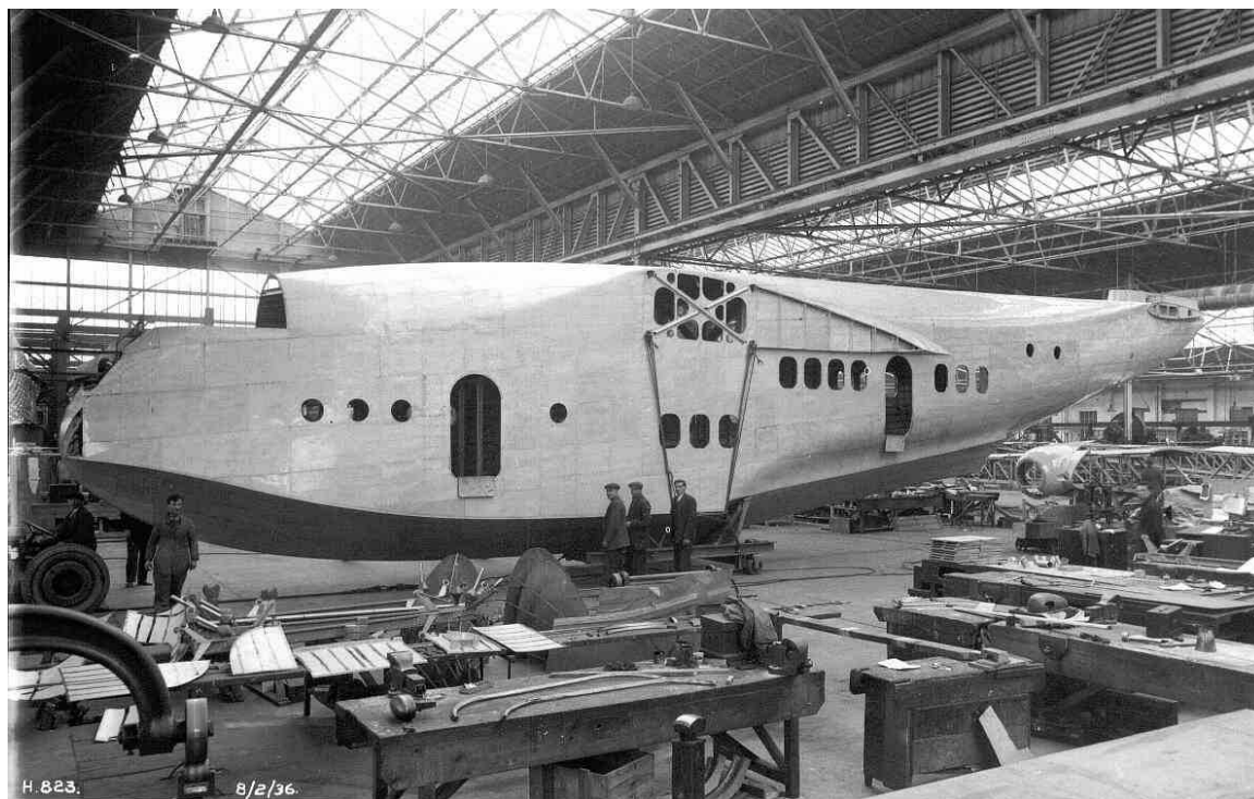
11. Short Bros. photo 832. 8 February 1936. The hull of the first Empire 'boat - minus the coup, but mated with the tail aft of Frame 42 - newly withdrawn from the gantry, perched on the shop truck. The hull has been turned on to the centre line of the main doors of No. 3 Shop with the nose pointing towards the main
